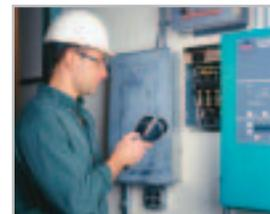
*Infrared can accurately and quickly locate faults before failures, shutdowns, or even fires occur.*
